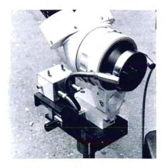
Stereo-zoom microscope which can be used with either 110 or 111 models of the Jensen Iriscope.
